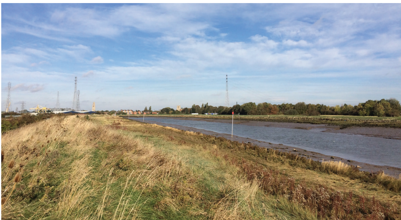
View of proposed wharf location
